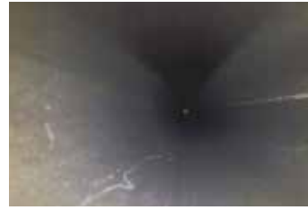
Figure 3. Evaporator tubing post treatment with Boss 302.
