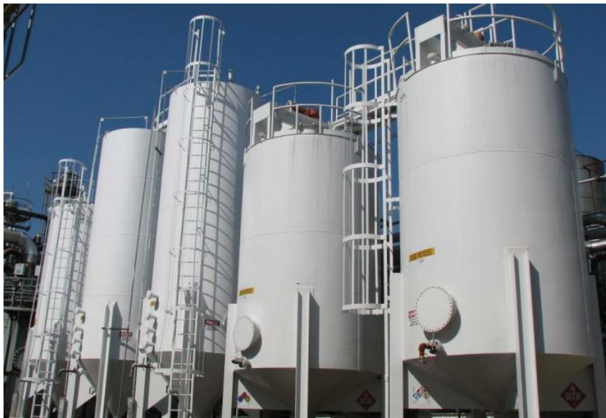
Storage tanks where carbon drums are often used to control emissions
